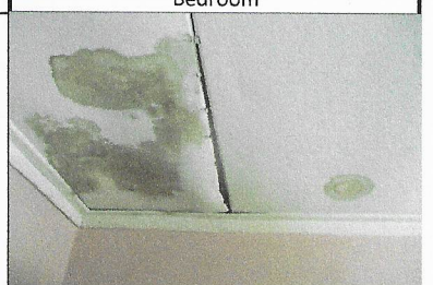
Roof leaks
