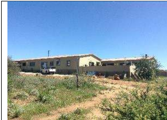
Main Building (MB)
